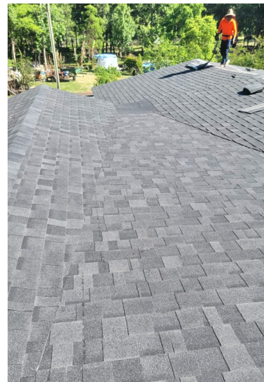
New roof installed after (Below)
